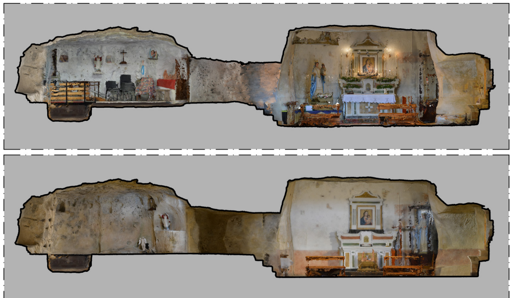
Fig. 7. Comparison of orthophotos of the Church of Madonna delle Vergini before and after restoration work. Graphic elaboration by the authors.
