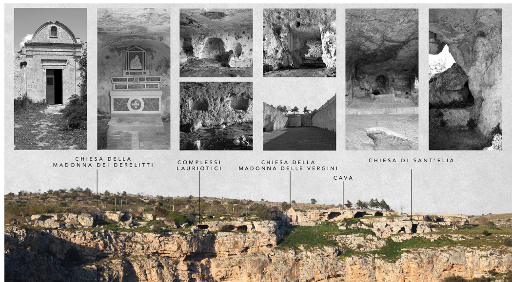
Fig. 3. Front view of Casale Sant'Elia and photographic details of its natural and anthropic marks. Graphic elaboration by the authors.
