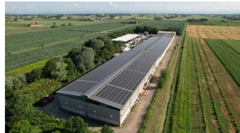
Composting plant Nonantola (MO).
