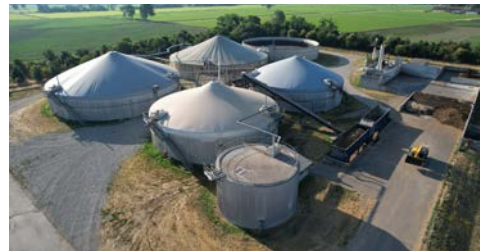
Agricultural biogas plant.
