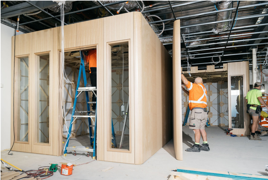
Fig. 16 - XFrame™ is a reconfigurable structural timber framing system that has been developed in response to the need to design buildings for change (Image courtesy of © XFrame™)
