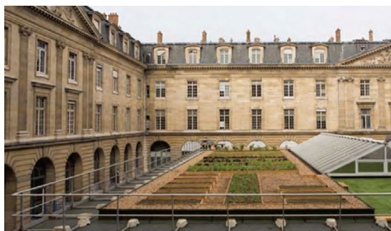
a. Green roof in an historical building in Paris center.
