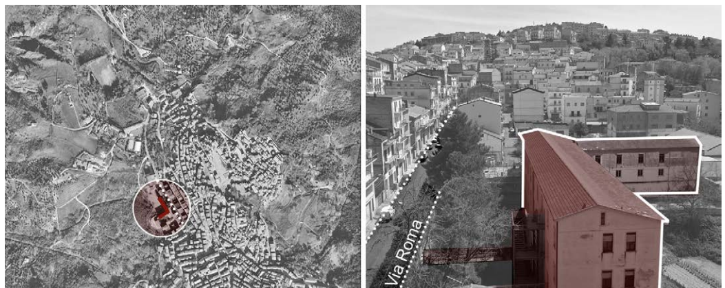
Fig. 3. Collage of images. Former school in via Roma in the urban center of Stigliano. On the left: framing orthophoto (Data source: Google Earth); on the right: aerial photo taken with a drone. Elaboration by the authors.
