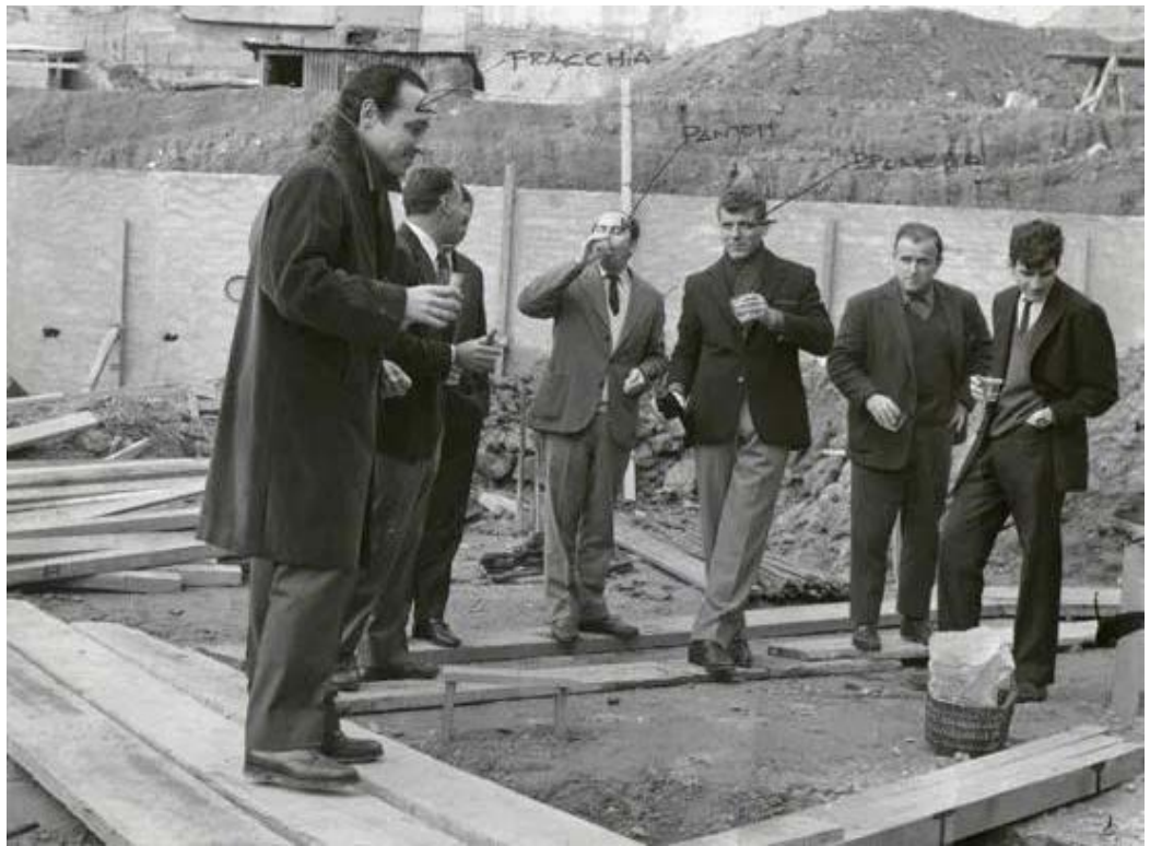
Fig. 2. Architectural members of Studio Pantoff-Fracchia during excavation at the beginning of work on the Olivetti Tower.
