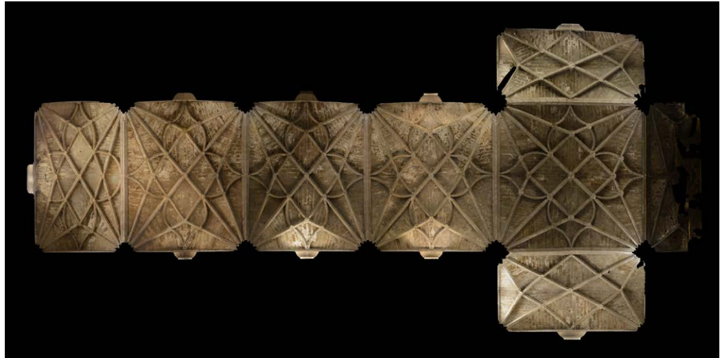
Fig. 5. Orthophoto of the intrados of the main vaulted system of the church of San Miguel, the model is sectioned above the jarjamento (graphic elaboration P. Borin).
