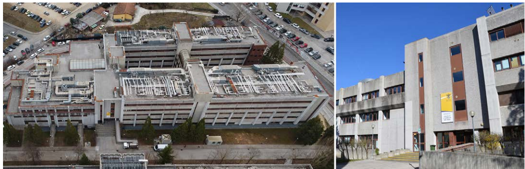
Fig. 1. The 'Angelo Camillo De Meis' building of the Coppito University Campus of the University of L'Aquila. Elaboration by the authors.
