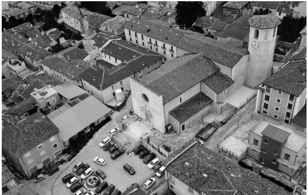
Fig. 1. Aerial view of the church and the square of San Pietro a Coppito. Elaboration by the authors.
