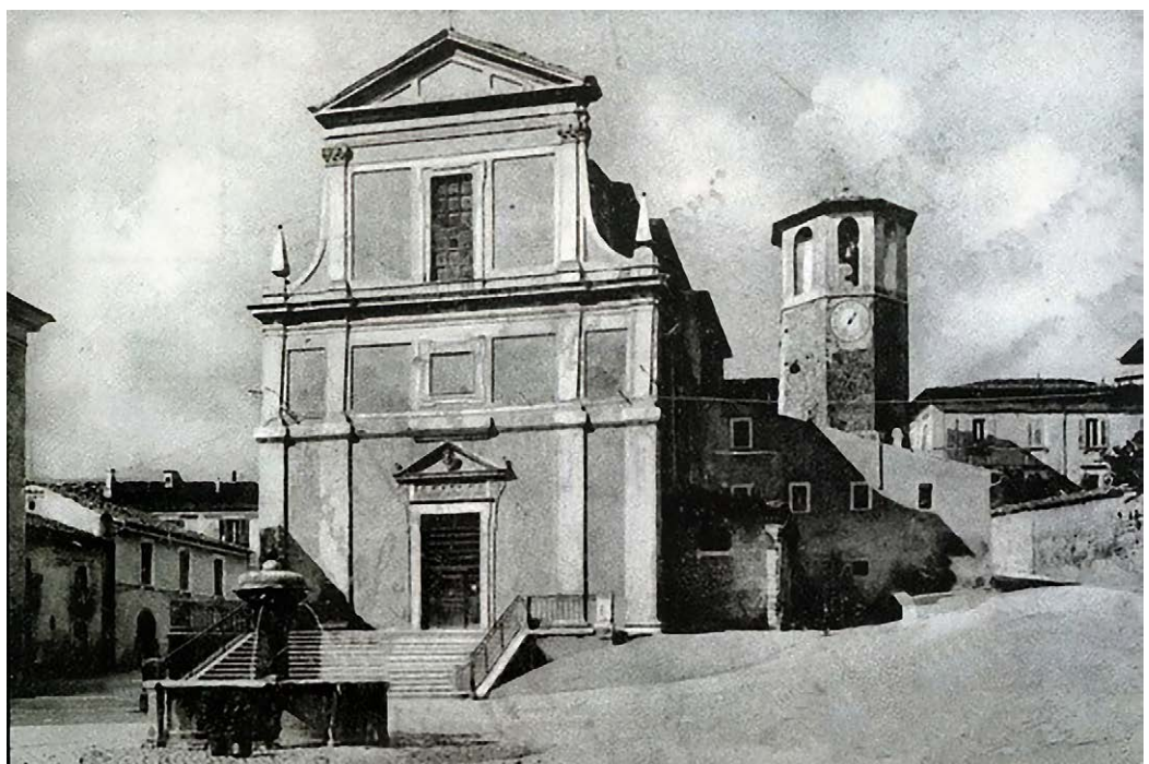
Fig. 5. The facade before the restoration of the years 1969-71.
