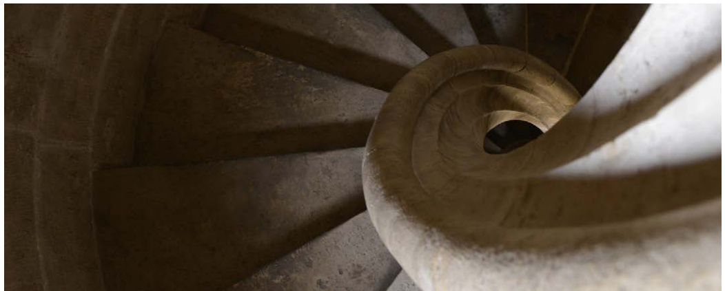
The helicoidal staircase of the tower of the Lonja de Valencia . Image by the authors.
