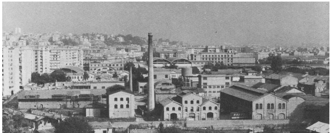
South View of the Former Mira Lanza Factory [L. Borroni, V. Giorgi 1976].
