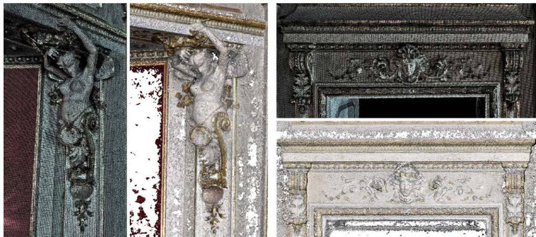
Fig. 9. Point clouds (laser scanner and photogrammetry) of some details of the decorative elements. Elaboration by the authors.
