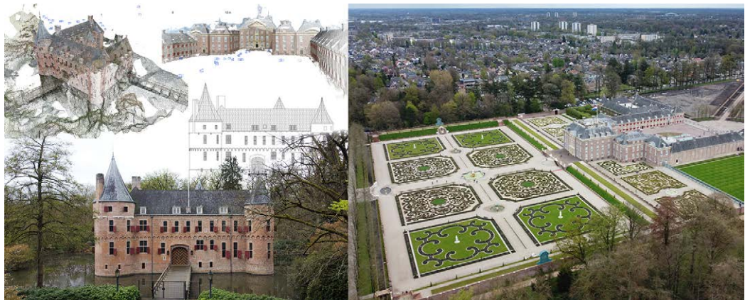
The royal residences of the House of Orange, workflow of the photogrammetric process, from point cloud to two-dimensional drawing. Elaboration by the author.
