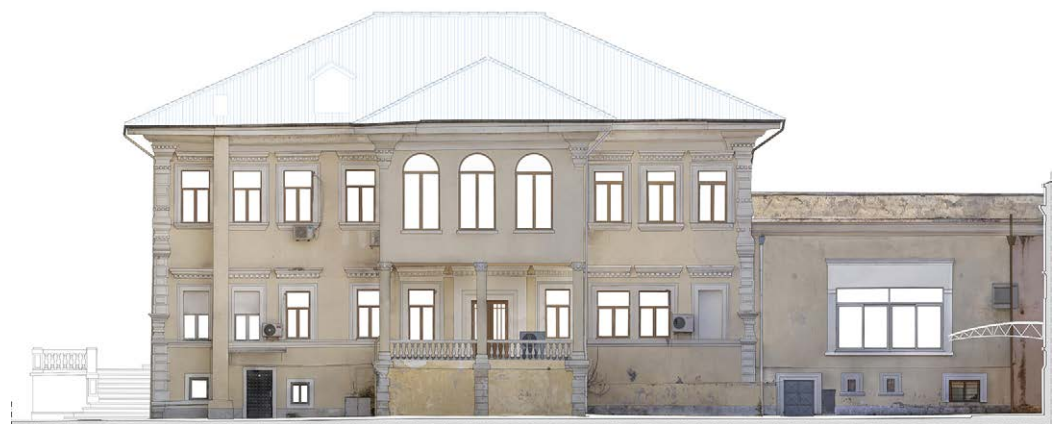
Fig. 6. Orthophoto of West Elevation. Elaboration by CHM_lab.
