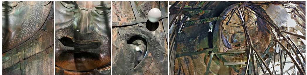
Fig. 4. Detailed images of the surface finish of the copper plates corresponding to the face of the Saint, highlighting the workmanship to achieve the "beard" effect. Elaboration by the authors.
