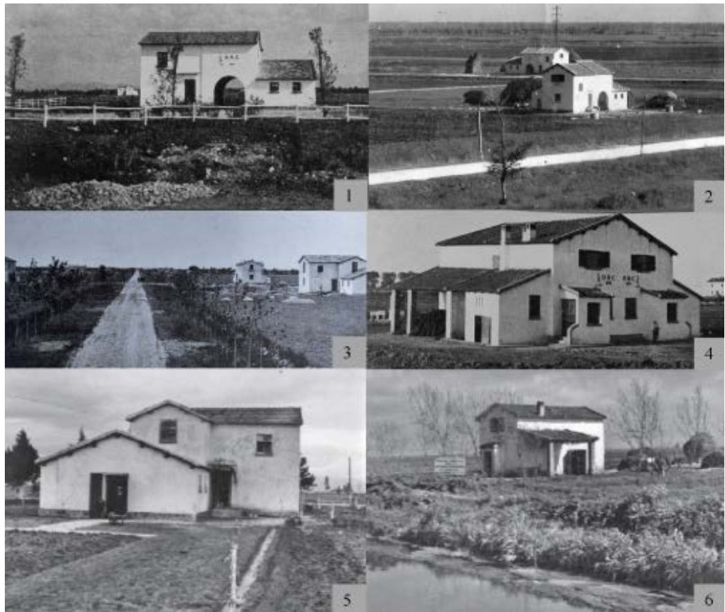
Fig. 3. Some period photographs: 3.1 Podere n. 26; 3.2 ONC-4056 photo [ACS]; 3.3 group of houses along the O. Salomone land reclamation road in Grazzanise; 3.4 house type V-E double ([AA.VV. 1955, p. 167]; 3.5 house type V-A ([Serraglio 2012, p. 148]; 3.6 house type V-E [Serraglio 2012, p. 148].
