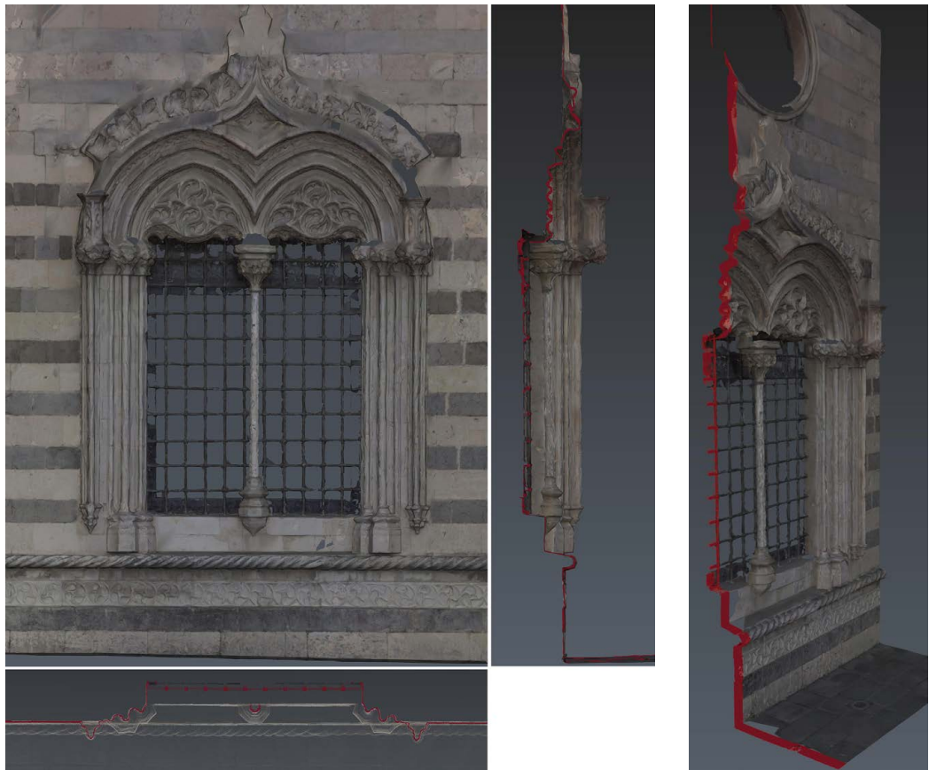
Fig. 4. Survey of the mullioned window of the Cathedral of Messina. Axonometric section. 3D model from the point cloud with mesh. Elaboration by the authors.
