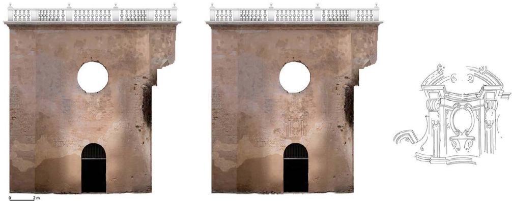
Fig. 7. Left: Orthophoto of the facade of the Church of Santa Maria della Grotta in Marsala. Center: Highlighting of the engraved design on the plaster. Right: Emphasis on the surviving traits of the perspective drawing of the portal. Elaboration by M. Cannella.
