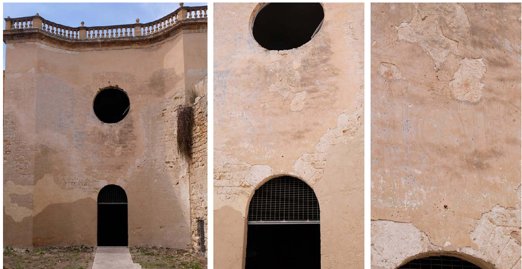
Fig. 4. Marsala. Complex of Santa Maria della Grotta, traces of the portal engraved on the facade of the church. Picture by M. Cannella.
