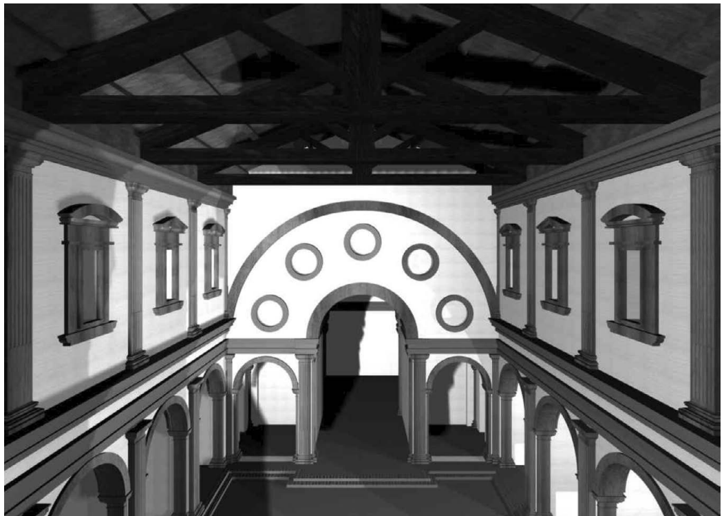
Fig. 11. Church of San Gallo. Reconstructive hypothesis of the interior; view towards the apse, trussed roofing, clerestory with decorative panel inspired by San Salvatore al Monte. Elaboration by Ylenia Ricci.
