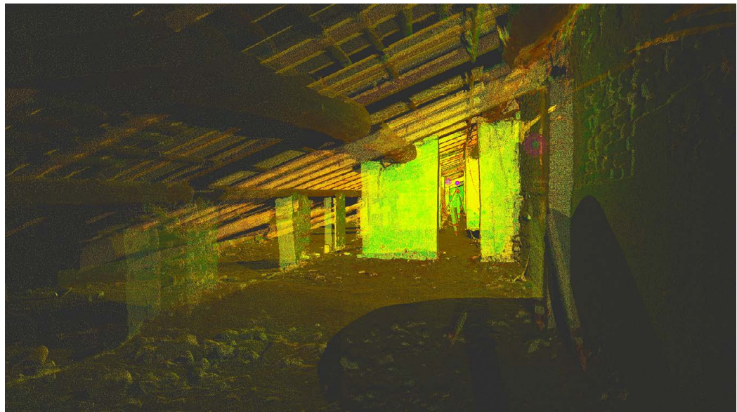
Fig. 8. Point cloud of tight and difficult-to-access roof spaces obtained from the laser scanner survey. Graphic elaboration by the authors.
