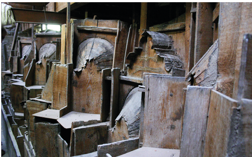
Fig. 1. The extrados of the ceiling (photo taken by the authors).
