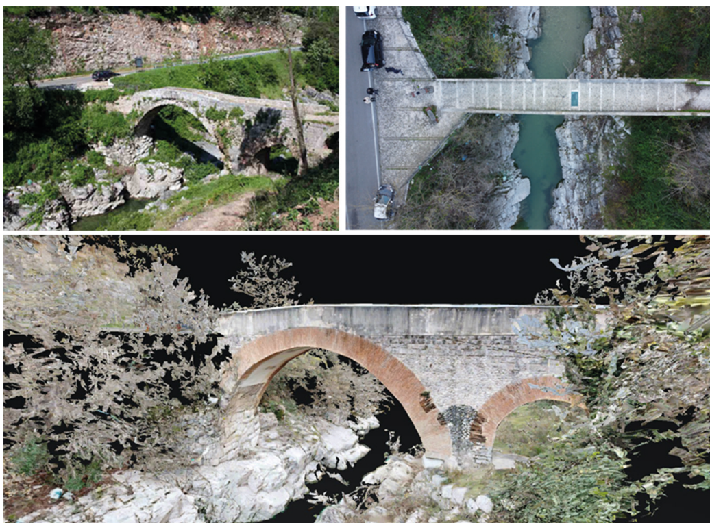
Fig. 5. Clockwise from top left: image prior to restoration; drone-based survey; laser scanning point cloud.
