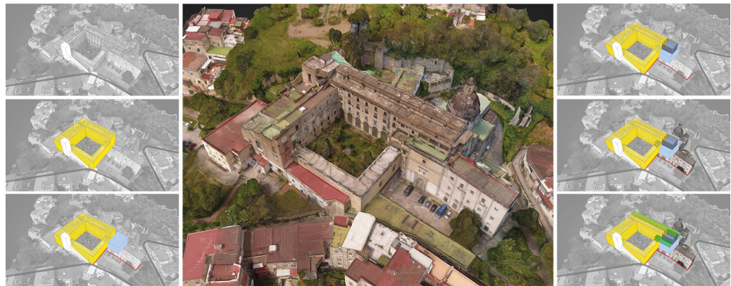
Fig. 2. Hypotheses of the architectural phases of the Santa Maria della Vita complex, from the sixteenth-century foundation plan to today (left and right), conducted on the basis of archive documents, integrated digital survey and textual documents (edited by V. Cirillo). In the center, a drone shot of the monastic complex (by R. Carrelli).
