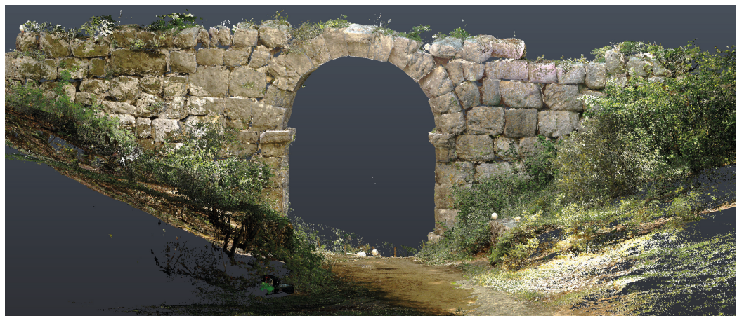
Fig. 2. Terrestrial Laser Scanning of the Trevi Arch (elaboration by authors).
