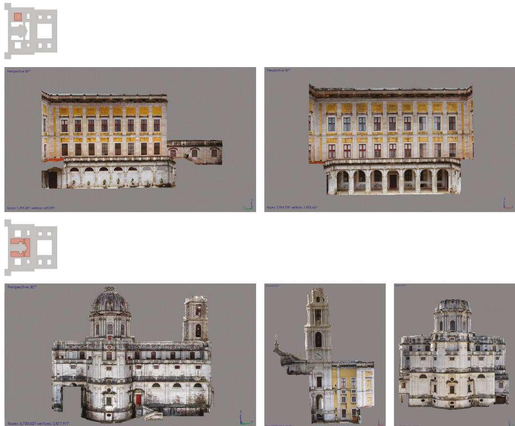
Fig. 2. Digital photogrammetric survey of the National Palace of Mafra. Above: Pátio do Rei; below: Cloister of the Basilica (elaboration by the authors).
