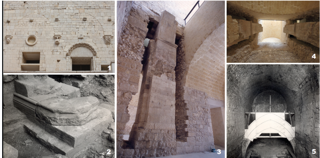
Fig. 5. Surviving elements of the north arcade: traces on the curtain wall of the ogival cross-vaulted ceilings and figured impost corbels (1); octagonal termination plinth on the masonry of the west wing (2). Surviving elements of the south portico: pillar incorporated into the backbone masonry of the 16th-century 'casemates' (3); archway after and during excavations, with evidence for the completion of the geometric layout (4), (5). Images courtesy of 'DRM PUG, Castello Svevo di Trani, TRANI (BT)' (image processing: authors).
