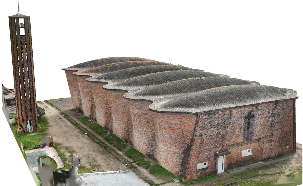
Fig. 5. Textured mesh model by photogrammetry (drone + terrestrial camera data, image by the authors).
