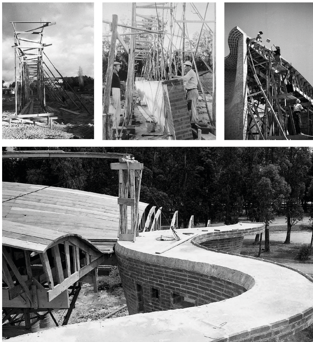
Fig. 1. Images of the construction site of the Church during the late fifties. Highlights are the interesting wooden ribs used to create the sinuous roof structure (Courtesy of Eladio Dieste Foundation).
