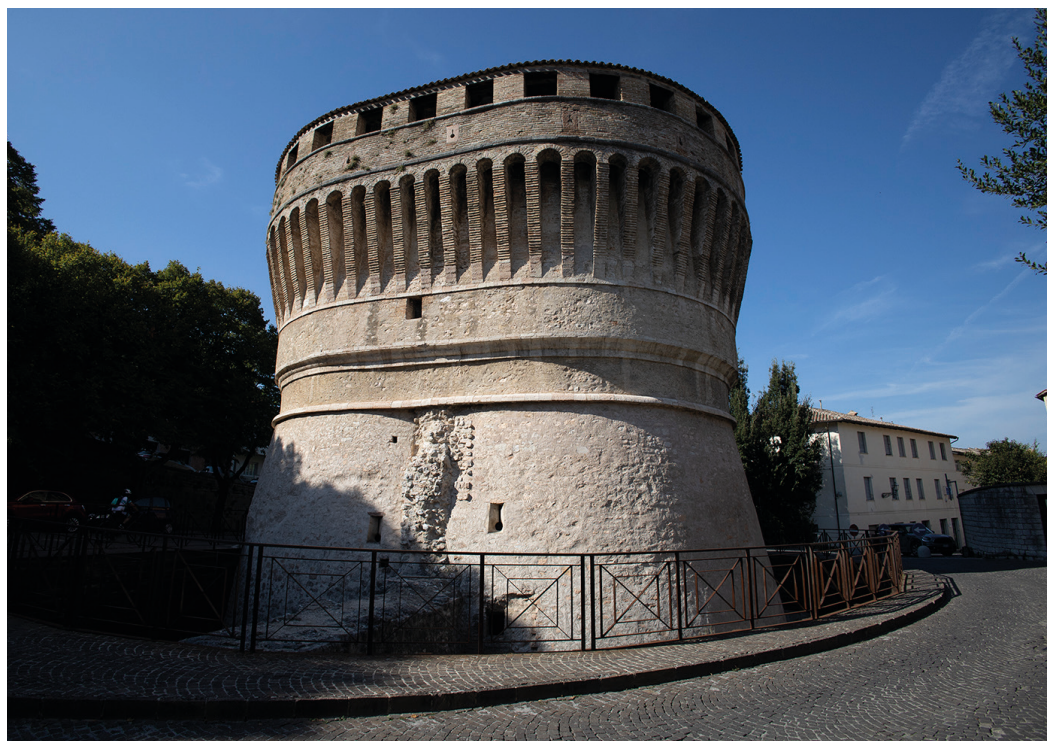
Fig. 5. External view of the Martiniana Tower; Center for Contemporary Sculpture, Cagli (Pesaro-Urbino) (photo by G. Galvani).
