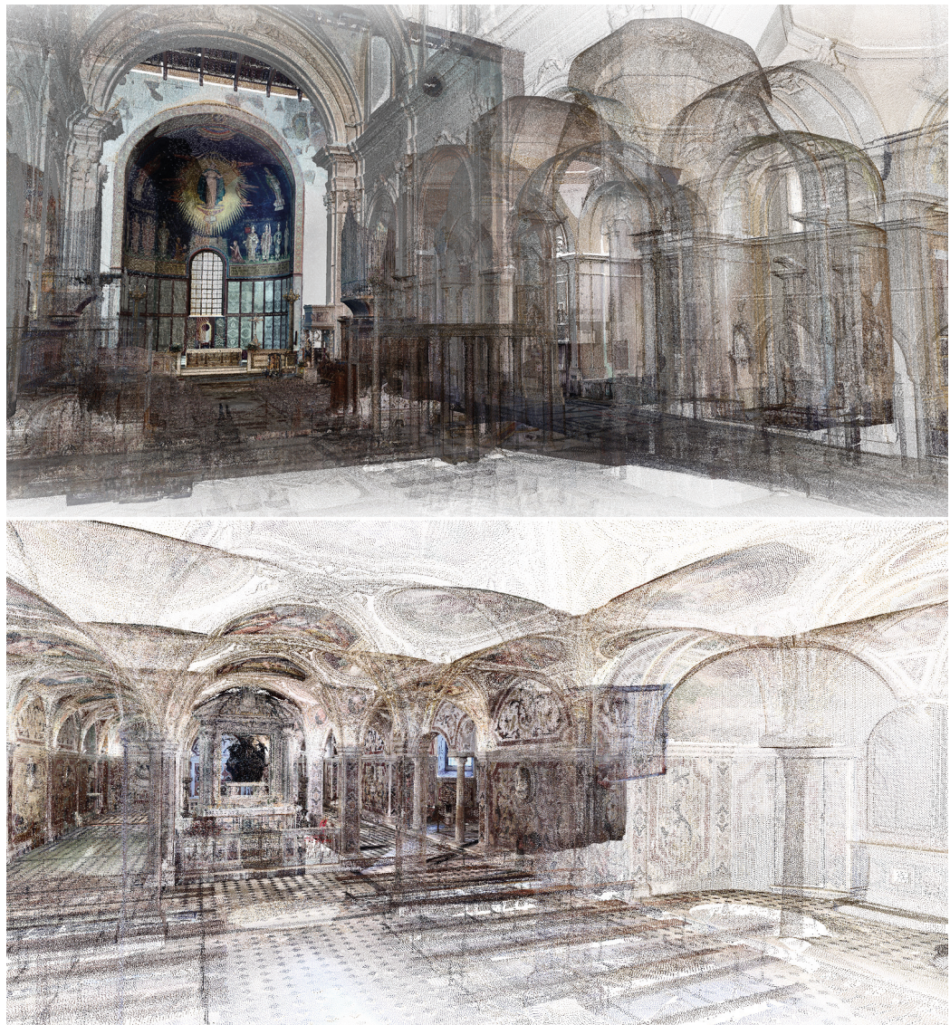
Fig. 3. Point clouds from terrestrial laser scanning of the interior of Salerno Cathedral (the upper basilica and crypt). Surveys conducted by the research group of the ModLab-Surveying and Geo-Mapping for Environment and Cultural Heritage, University of Salerno (June 2024).
