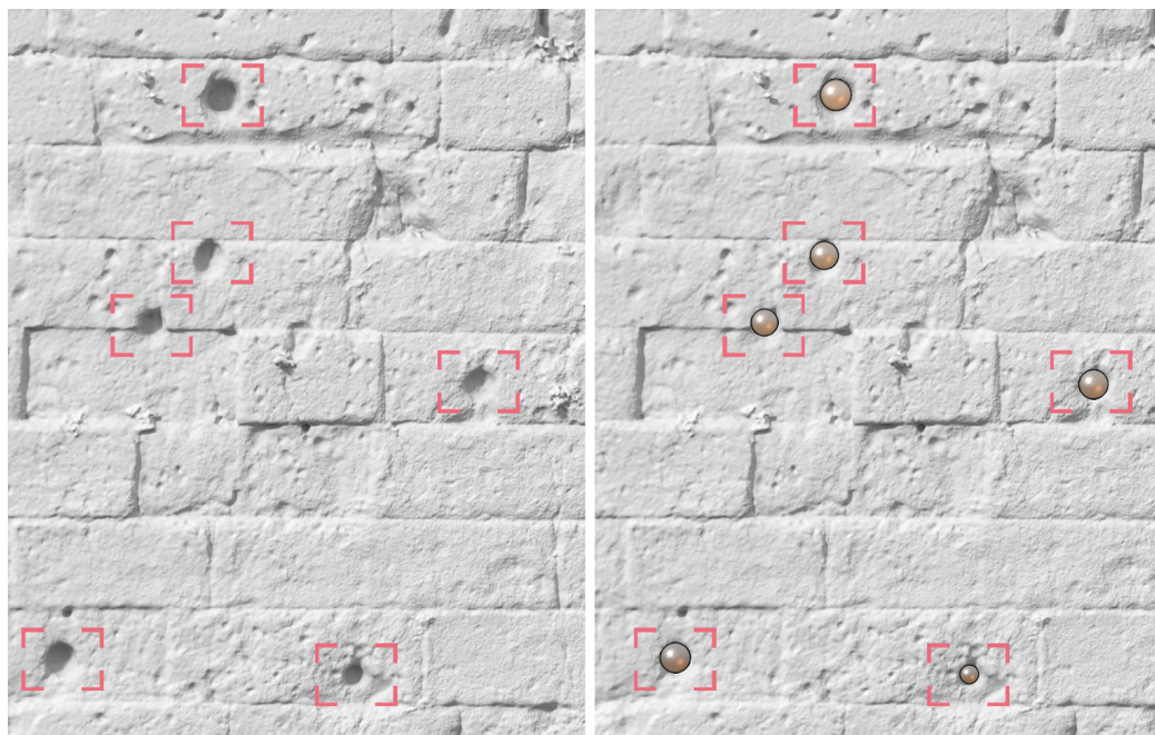
Fig. 3. Examples of ballistic marks documented on the stretch of the city walls near Vesuvio Gate and the corresponding impacting projectiles (models by S. Bertacchi).
