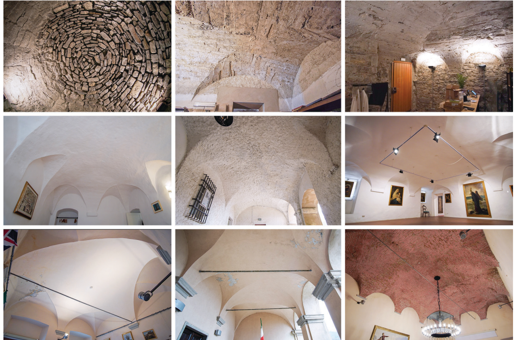
Fig. 2. Selected examples of the types of vaults present in the castle (elaboration by the authors).
