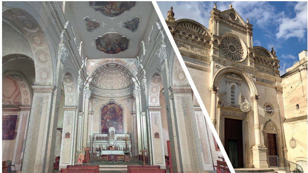
Fig. 1. The Church of Saint Mary Veteran in Triggiano. Left: point cloud of the internal structure; right: main façade of the church (elaboration by the authors).
