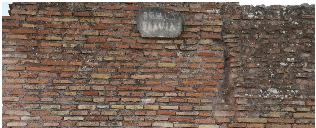
East wall in Opus Testaceum of the triclinium in the Domus Flavia on the Palatine Hill (photo by the Author).
