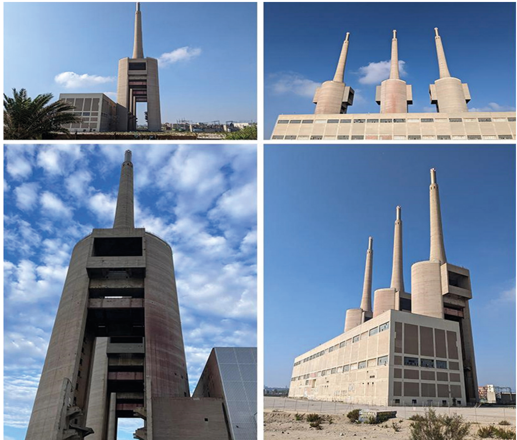
Fig. 1. Thermoelectric power station of Sant Adrià de Besòs, Spain (photographs by M. Proietti and F. Zollo).
