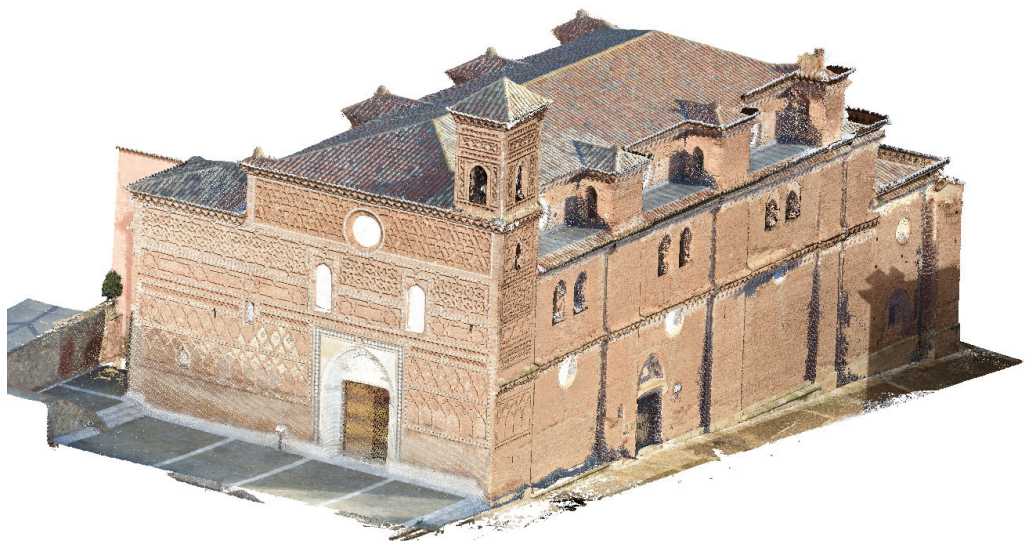
Fig. 2. Point cloud obtained by drone photogrammetry of the Church of Santa María de Tobed (own elaboration).
