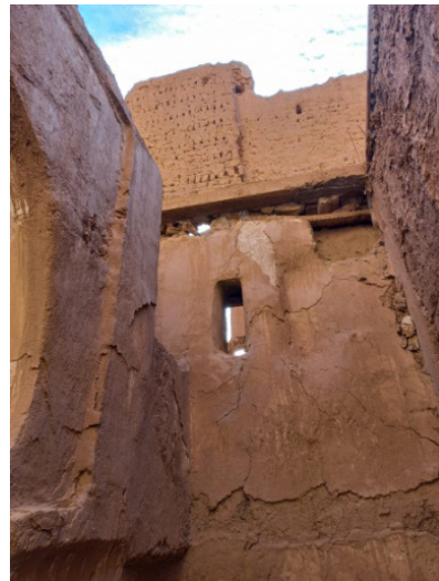
Figure 23 - Surface detachment of the earthen mortar
