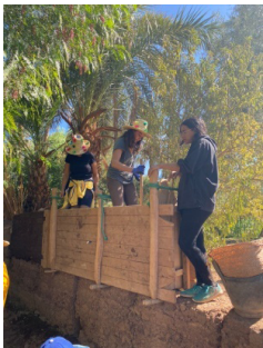
Figure 15 - Students using azduz during the Construction of the wall, author 2021
