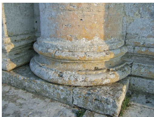
Figure 15 - The figure shows a growth of yellowish lichens on the travertine architectural decorations of the Church of San Biagio in Montepulciano (credits Oana Adriana Cuzman)
