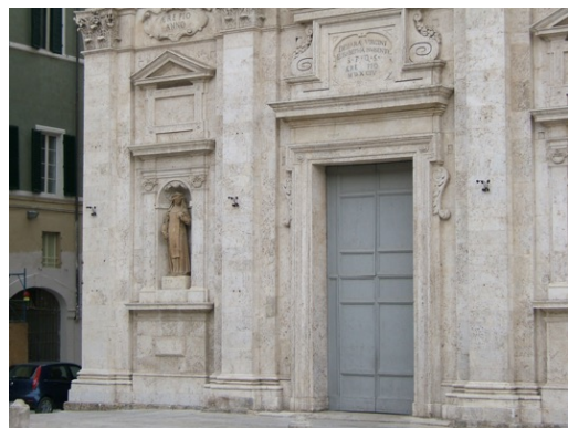
Figure 4 - The figure shows the travertine cladding of the façade of the church of Santa Maria di Provenzano in Siena (17 th century). The façade is divided into three parts by pilasters, divided into two levels by a cornice and culminating in a tympanum. In the centre, the portal is surmounted by an arched tympanum and a rectangular window, while on either side there are four niches with statues of Saints Ansano, Vittore, Caterina and Bernardino (credits Fabio Fratini)
