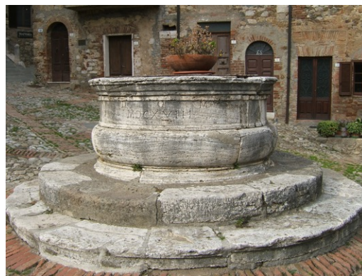
Figure 7 - The figure shows a travertine well dating back to 1618 in Castiglione d'Orcia (province of Siena). The well is located in Piazza Vecchietta, a triangular-shaped square on a slope paved with cobblestones enclosed in squares formed by rows of bricks laid on edge that converge towards the well (credits Fabio Fratini)
