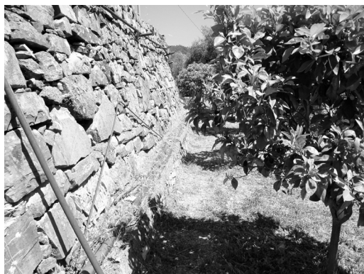
Figure 10 - Vallebona (IM): the little channel at the base of a drystone wall, occupied by the new pipes to water the citrus groves
