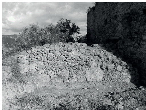
Figure 15 - Dry structure made with recycled materials
