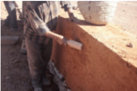
Figure 16 - Maâlem, stripping the wall, author 2021
