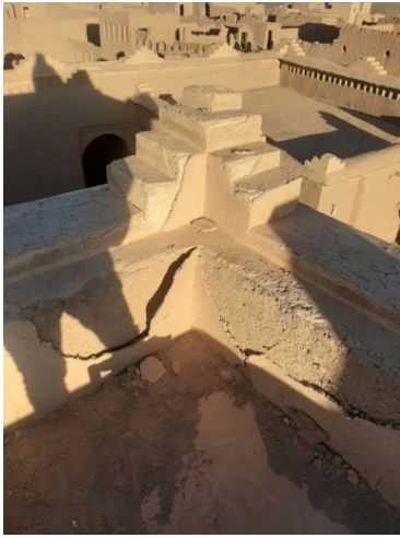
Figure 24 - Surface detachment of the earthen mortar, author 2001 and craks, author 2021
