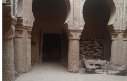
Figure 26 - Degradation of the base of a column, author 2001
