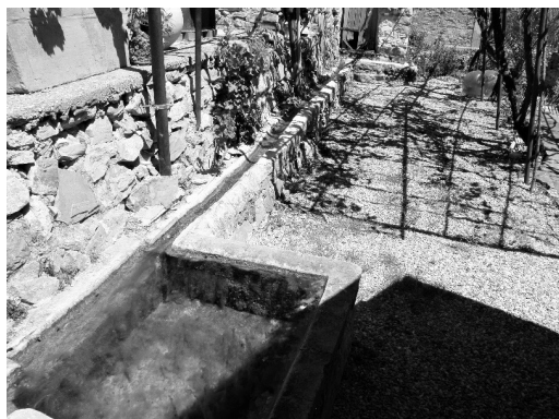
Figure 4 - Vallebona (IM), channel and water collection tank.
