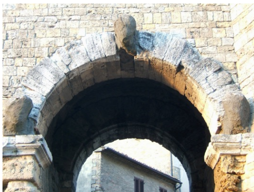
Figure 3 - The figure shows Porta dell'Arco, the main entrance gate on the southern side of the Etruscan walls of Volterra. This gate features a round arch made of well-squared blocks of travertine. At the keystone and the two imposts, there are three heads carved in a volcanic rock from Montecatini Val di Cecina, hardly legible due to severe deterioration (credits Fabio Fratini)
