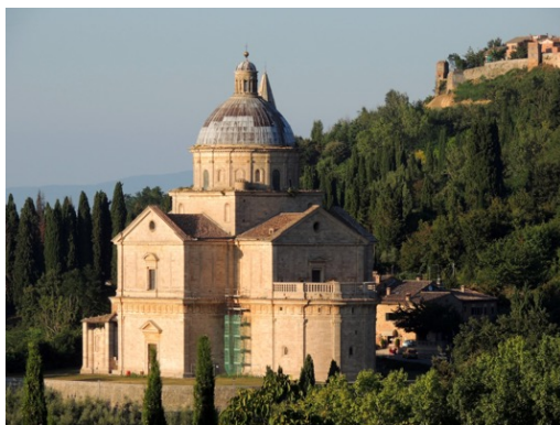
Figure 8 - The figure depicts the church of San Biagio in Montepulciano, a fine example of 16 th century Renaissance architecture, entirely clad in travertine. The Greek cross plan with a central dome set on a terrace and a classical drum is visible (credits Fabio Fratini)
