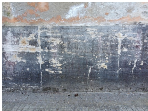
Figure 14 - The figure shows a dark grey biological colonization in a travertine baseboard (credits Oana Adriana Cuzman)
