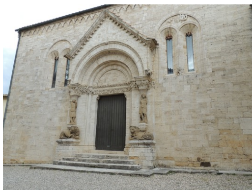
Figure 6 - The figure shows the south side of the Church of Saints Quirico and Giuditta (12 th -13 th century) in San Quirico d'Orcia (province of Siena) clad in finely hewn whitish travertine ashlar. There is a Lombard-style portal (13th century) supported by two caryatids resting on two lions, all in Pliocene sandstone (credits Barbara Sacchi)
