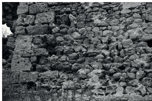
Figure 9 - Detail of a masonry with a cantonal corner in puddinga
