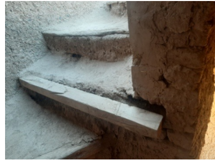
Figure 25 - Detachment of retaining boards of stairs
