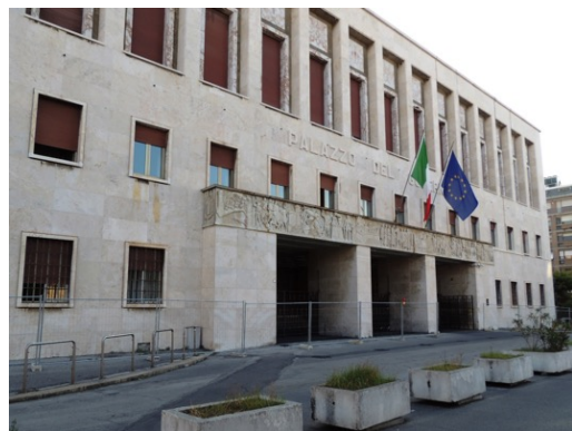
Figure 11 - The figure shows the rationalist façade of the Government Palace in Livorno, clad in travertine (credits Fabio Fratini)
