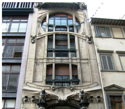
Figure 13 - The figure shows an image of the Casa-Galleria Vichi in Florence, an Art Nouveau building covered in artificial travertine (credits Fabio Fratini)
