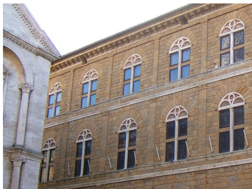
Figure 5 - The figure shows the façade of Palazzo Piccolomini in Pienza (15 th century) with its façade in finely hewn Pliocene sandstone of ochre colour and window frames in whitish travertine. On the left is part of the Cathedral façade, with its whitish travertine cladding (credits Barbara Sacchi)
