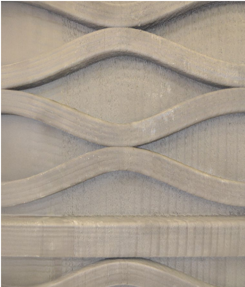
Figure 17. 3D printed hollow ribs structure.
