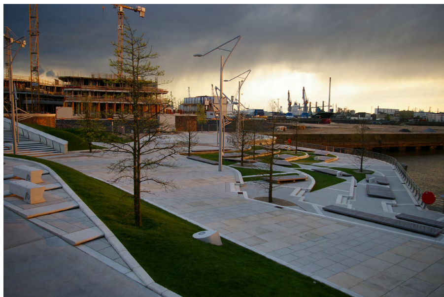
Fig. 2 - Hafencity public spaces by Miralles/Tagliabue, Hamburg. Photo by Marco Polo Terrassen.
