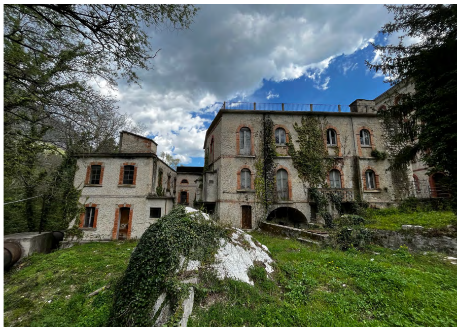
Fig. 3 - The former Cipolla Wool Mill in Fara San Martino. Photo by Massimo Angrilli.
