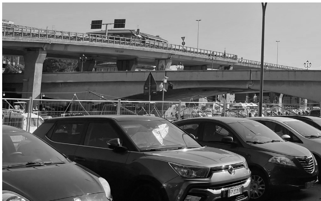
Fig. 6 - Ponte Risorgimento and the parking lot. Photo by Lorenzo Morelli. [5]
