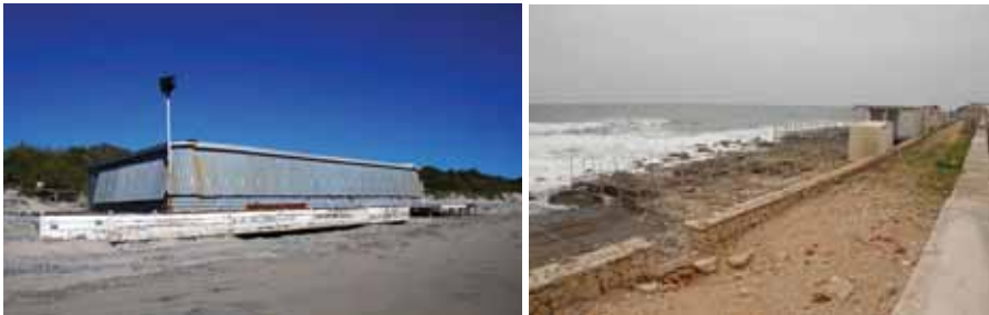
Figg. 05, 06 : Bathing facilities during the winter shut down in a state of abandon and neglect
