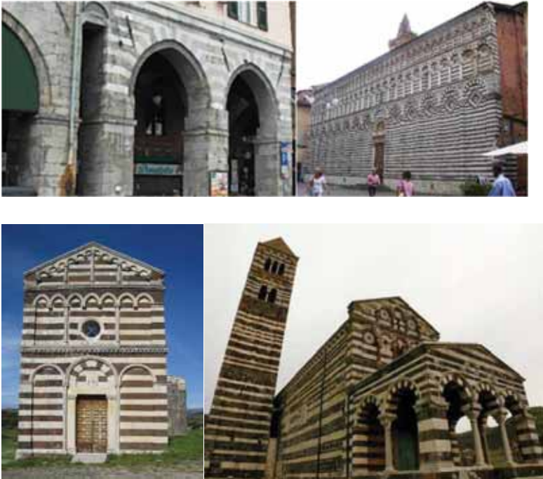
Fig. 04 : The alternating voussoirs or bichrome stripes of white and black: (b2) Ripa maris, an arched infrastructure with a commercial function; (c) Pistoia, church of San Giovanni Evangelista, known as San Giovanni Fuorcivitas ; (d) Bulzi (Sassari), San Pietro del Crocifisso, and Codrongianos; (e) Sassari, Basilica of the Holy Trinity of Saccargia
