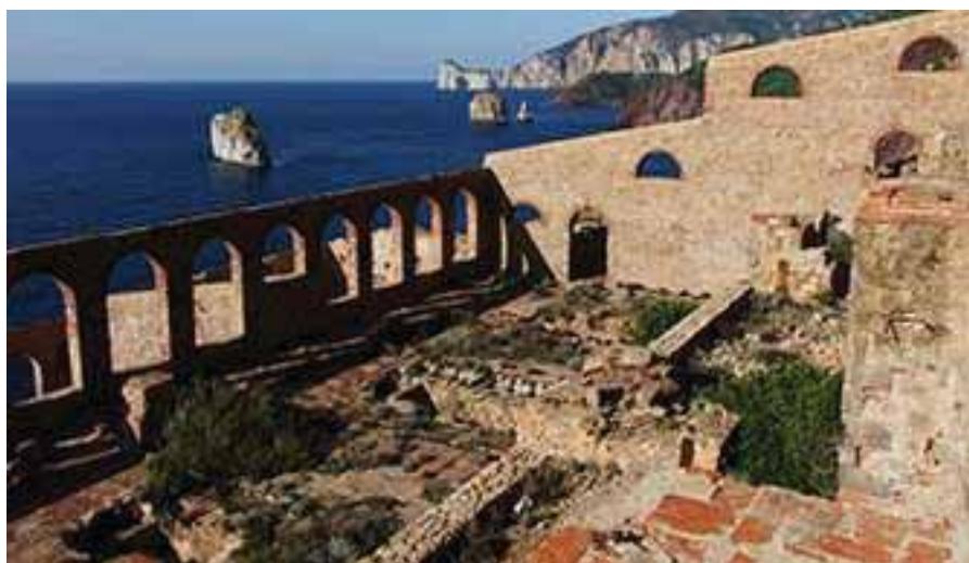
Fig. 06 : Interior view of the laveria
