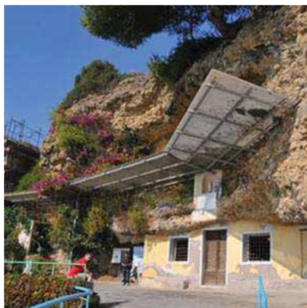
Fig. 03 : The sanctuary from the outside
