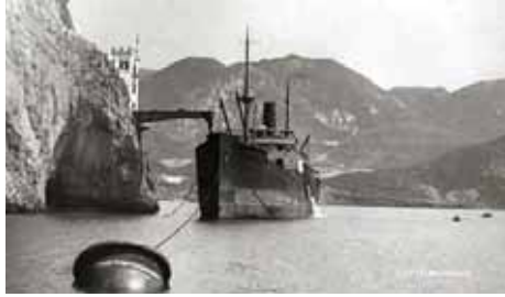
Fig. 01 : Loading of the mineral ore onto the steamships using the mechanical swivel arm overhanging the sea, Igea Archive, Iglesias
