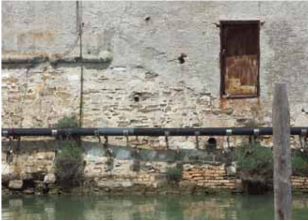
Fig. 02 : Graft between the wall of the bastion and the new construction
