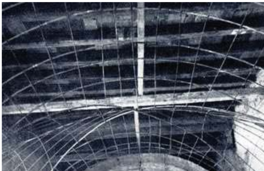
Fig. 08 : Metal frame of hanging vaults
