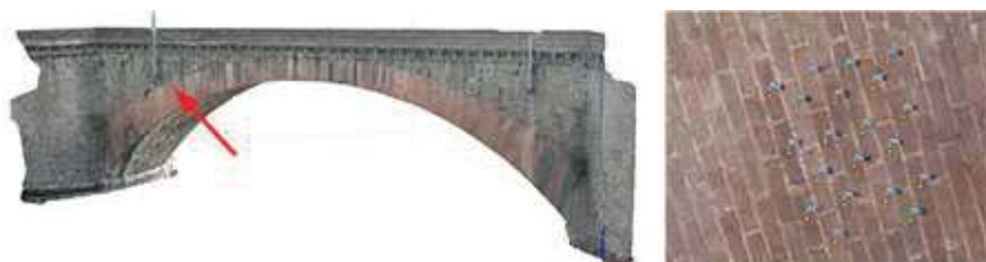
Fig. 03 : Case B. Tiled view of Prarolo bridge 3D model and marked bricks
