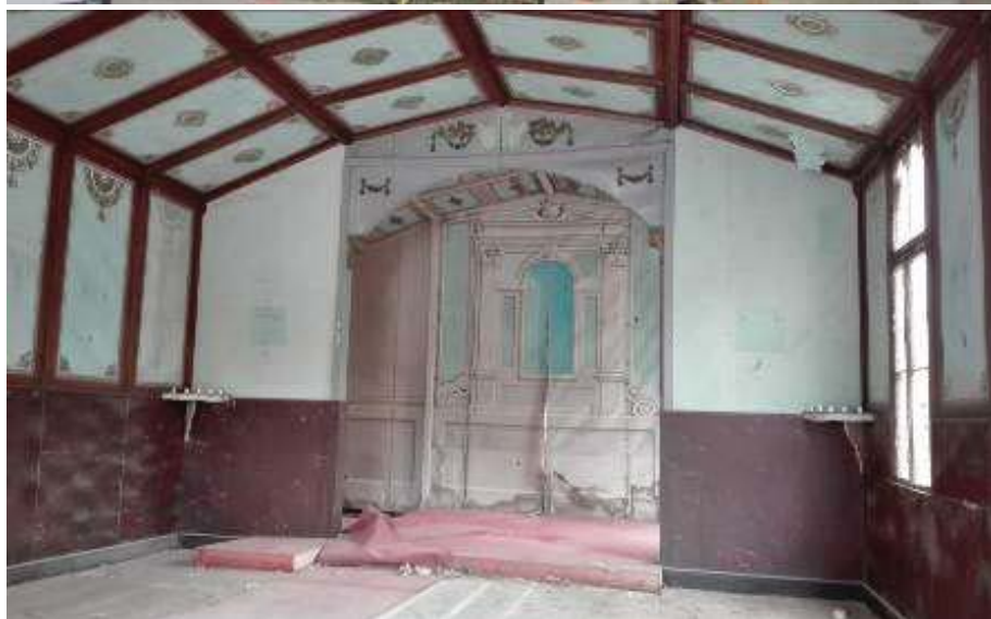
Figg. 03/04 : Cappella di Fegino (Genova), outside view (03) and internal view (04)
