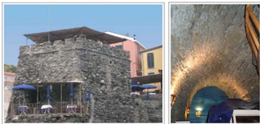
Fig. 03 : Internal and external of Belforte
