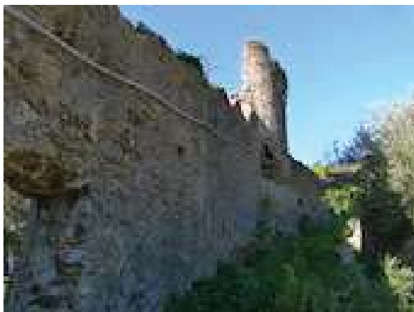
Fig. 10 : The tower and the walls
