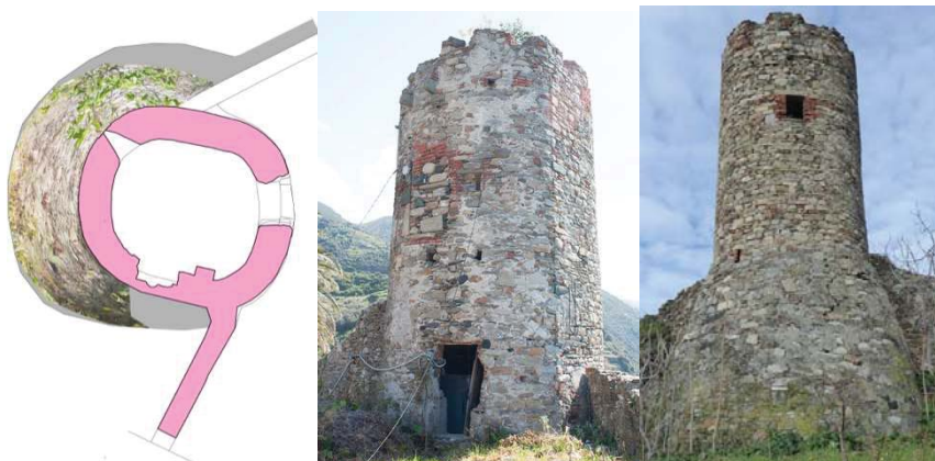
Fig. 03 : From the left: plan of the tower at 1.60 m above the entrance level (41.60 m above sea level); side view: notice the vertical junction between the oldest and the most recent part; side facing the sea
