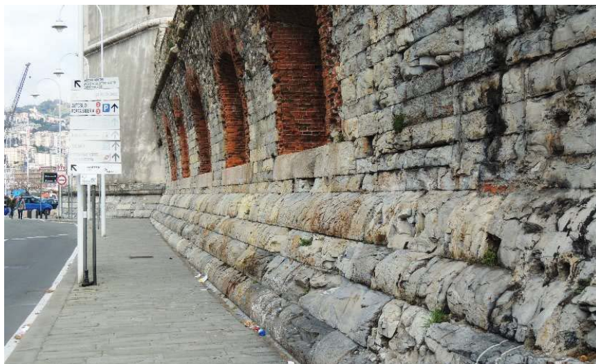
Fig. 07 : Ashlars in marly limestone in the pier walls near Porta Siberia in the pier
