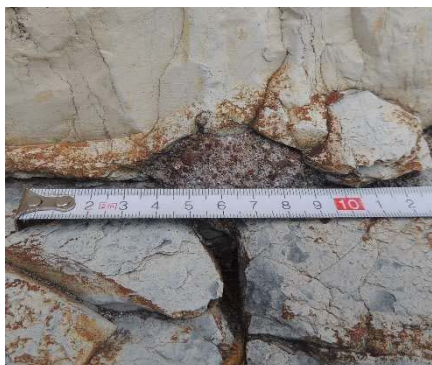
Fig. 10 : Bedding mortar of the pier walls near Porta Siberia with pozzolana (sample 6)
