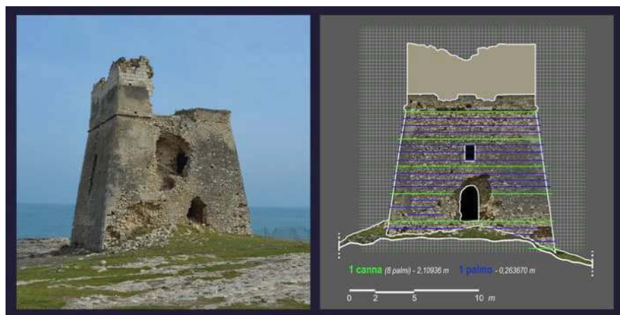
Fig. 02 : Sfinale Tower. Masonry horizontal alignments of the South side
