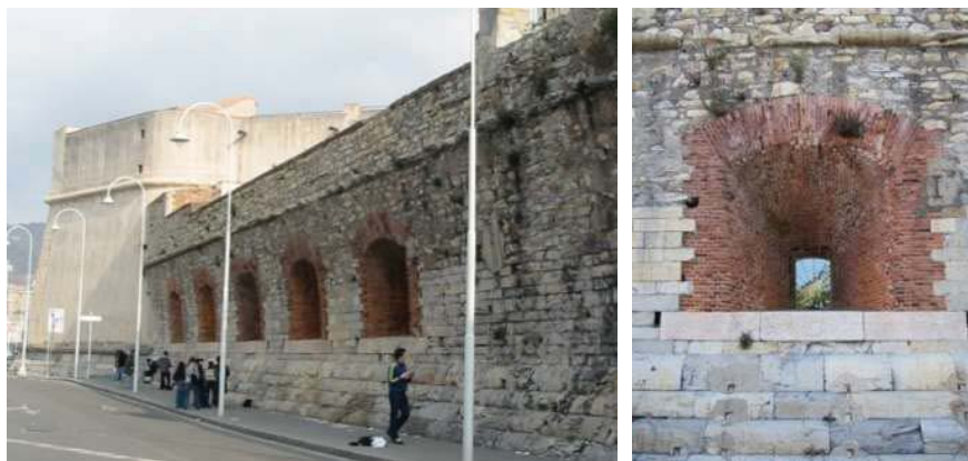
Figg. 15a, b : The Battery in 2006, during the educational exercise: part facing the sea (a) and detail of a cannon embrasure (b)
