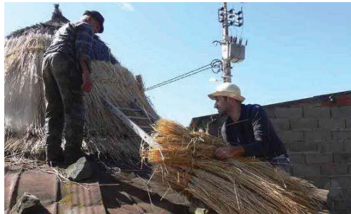
Fig. 10 : Corte de Ouro, placing the rye straw on the cover (Pinto, 2015)
