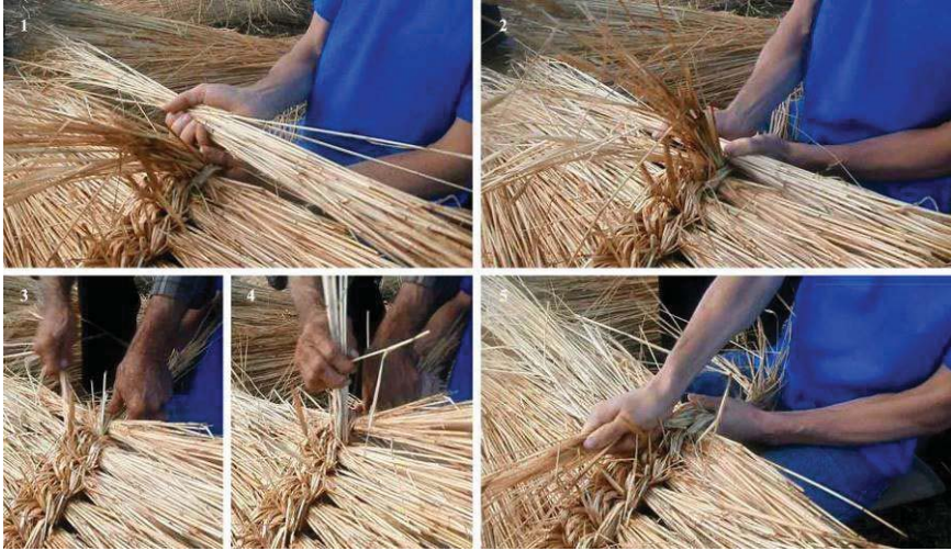
Fig. 09 : Corte de Ouro, process of weaving rye straw (Pinto, 2015)
