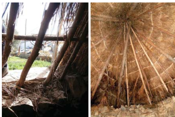
Fig. 04 : Corte de Ouro, haystack. Left side : top of the wall. Right side : interior of the conical dome (Pinto, 2015)
