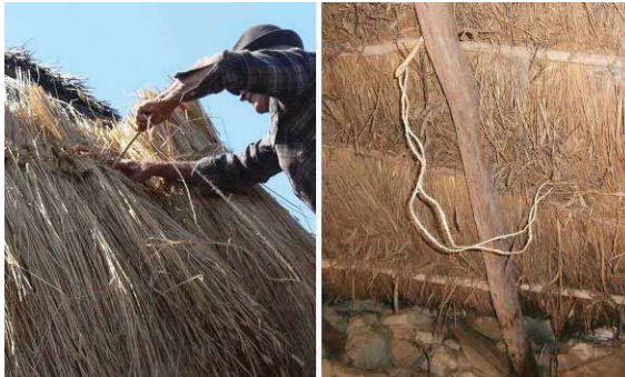
Fig. 06 : Corte de Ouro, sewing of the braids of rye straw. To the left : exterior view of the roof. To the right : interior view of the roof (Pinto, 2015)
