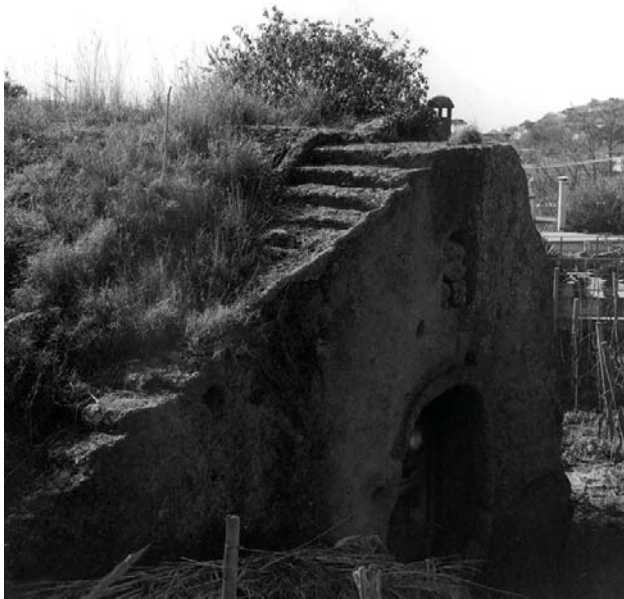
Fig. 05 : F. Castiglione, Exterior staircases of a stone-house in Panza, Forio
