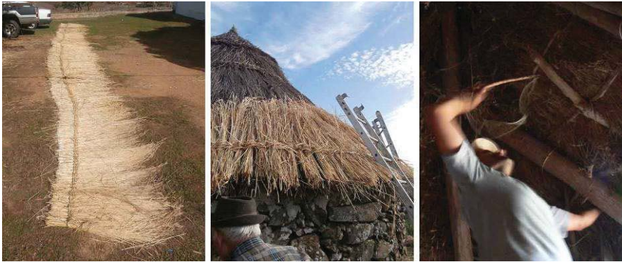
Fig. 05 : Corte de Ouro, Tavira. From the left side to the right : preparation of the haulm (Pinto, 2015); placement of the stalk on the canopy with the process of reinforcement (Pinto, 2015) ; stitching process (Pinto, 2015)
