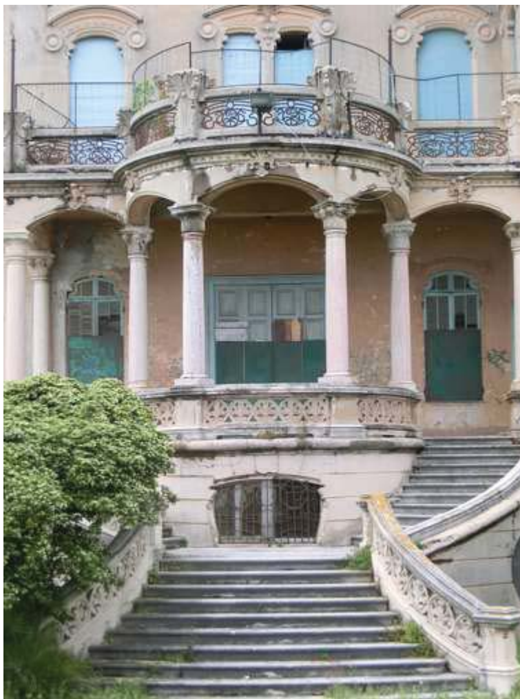
Fig. 03 : Detail of the portico on the seafront of Villa Zanelli
