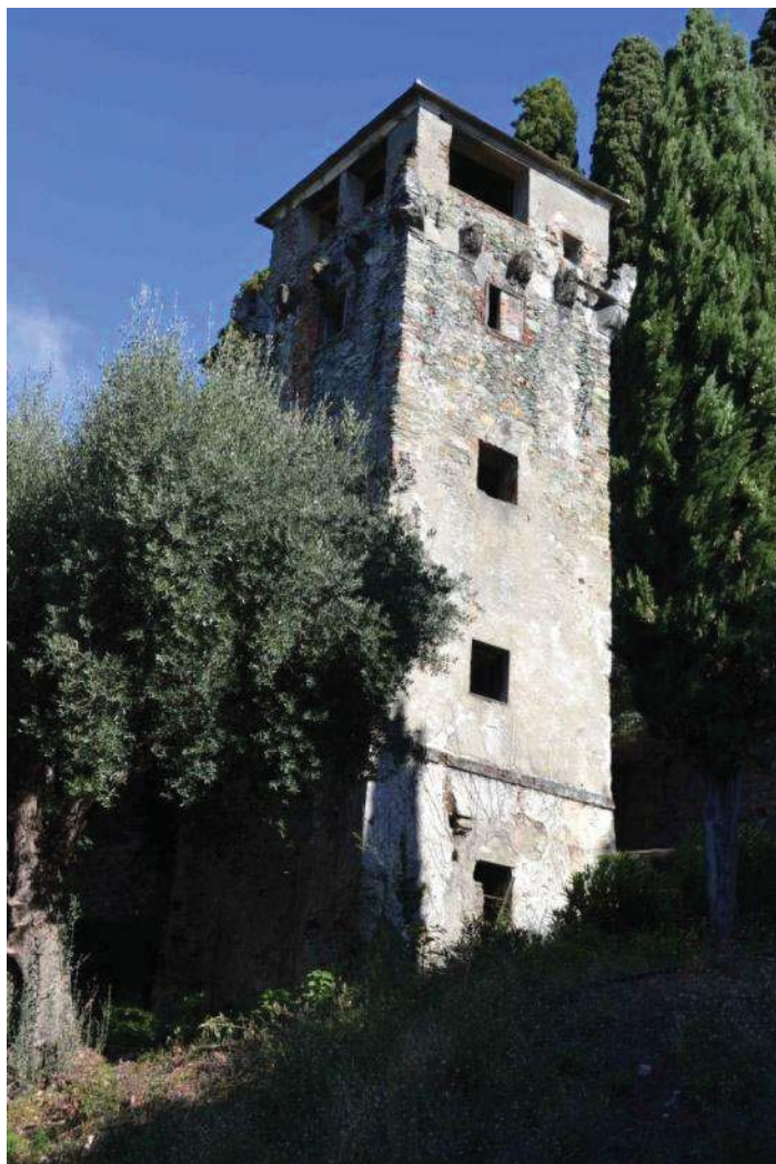
Fig. 02 : Exterior view of the southwest corner of the "Saracen tower"
