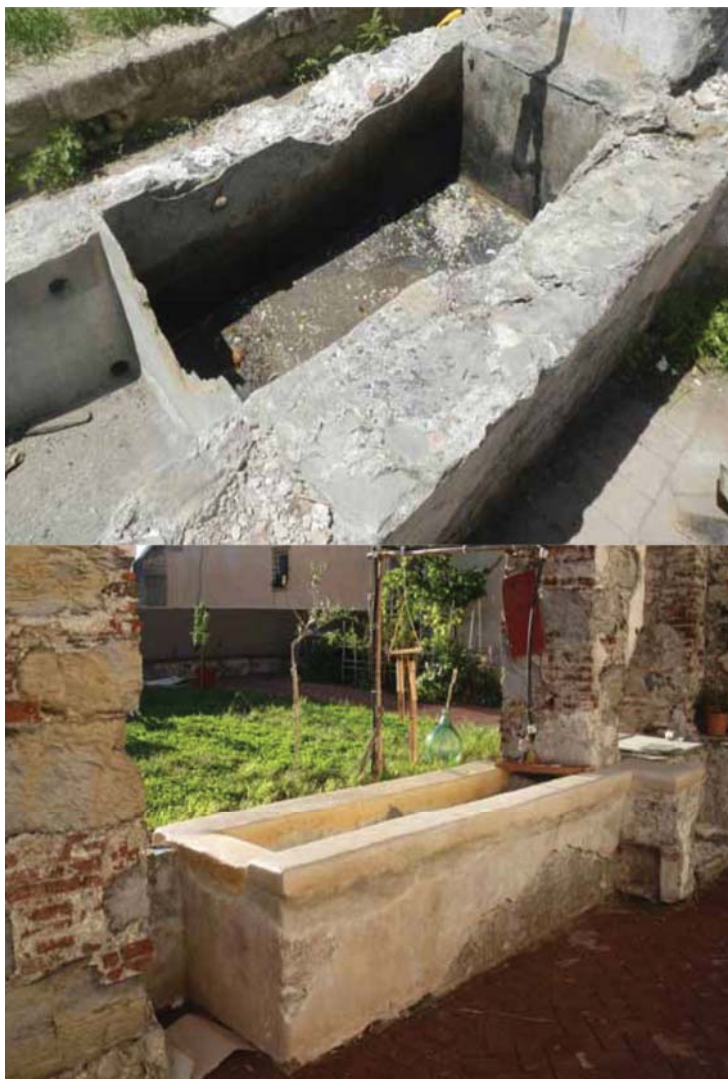
Fig. 03 : The conditions of the washhouse tubs of the monastery before and after the intervention
