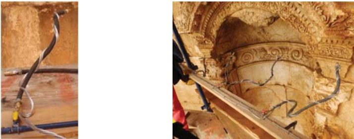
Fig. 01 : Trials of building nebulisation equipment with rubber pipe
