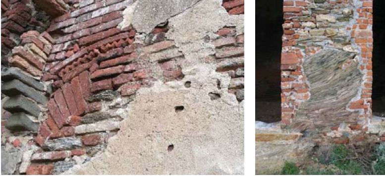
Fig. 05 : Modifications in the oldest part of the tower (photo by the authors). Fig. 06 : Pillar carved into the rock and rectified with bricks (photo by the authors)
