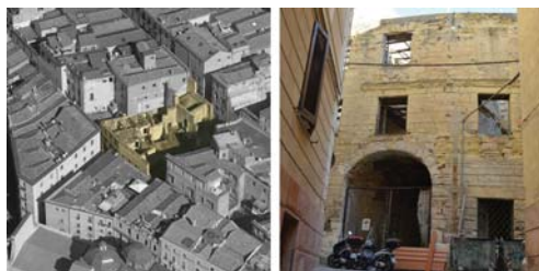
Fig. 01 : Localisation and façade on Via dei Genovesi of the Aymerich Palace
