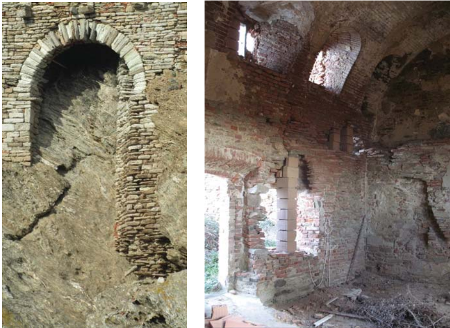
Fig. 07 : Loss of lithic material at the base of the discharge arc (Photo by the author). Fig. 08 : Decay phenomena in the internal rooms of the tower (photo by the authors)
