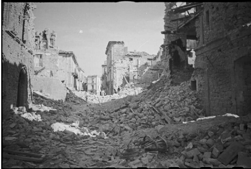
Fig. 3 – Section of the ruins of the town of Orsogna, Italy, World War II - Photograph taken by George Kaye.- Fonte: PAColl-4161: New Zealand DA-06278-F. Alexander Turnbull Library, Wellington, New Zealand.
