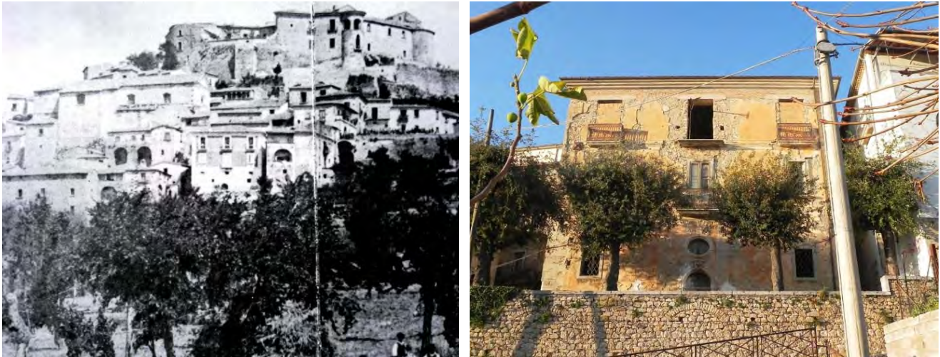
Fig. 2 – On the left: 19 th -century South view of the old town, with the castle and its curtain walls on top, the mother church on the left, and Palazzo Dell'Erario in the lower middle; the openings at the basement had not still enlarged – Source: Grappone & Iannarone, 2009. On the right: Current view of the main façade of Palazzo Dell'Erario from the foot of the city wall remains
