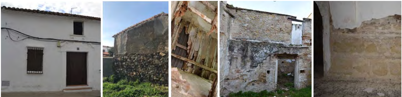
Fig. 2 – Materials and constructive solutions recognized in some locations - Source: Carrascosa Gómez, Plaza Bermejo “(Plaza, 2017)”
