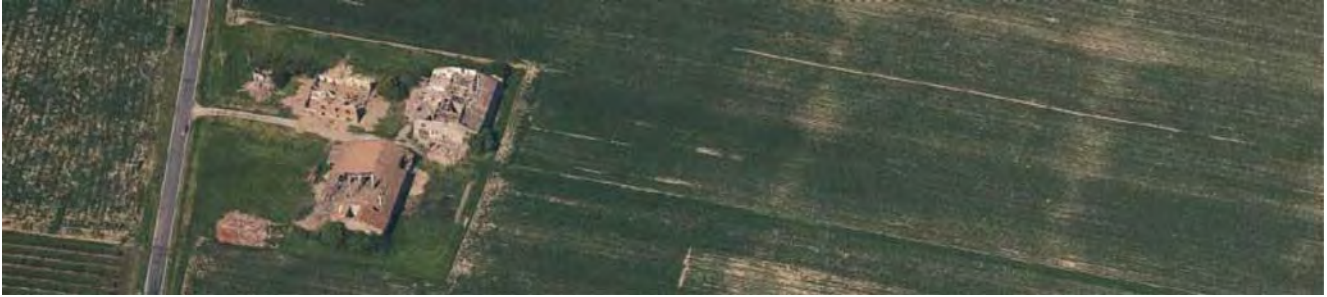
Fig. 3 – Mirandola (MO), the damage scenario of a historic courtyard.
