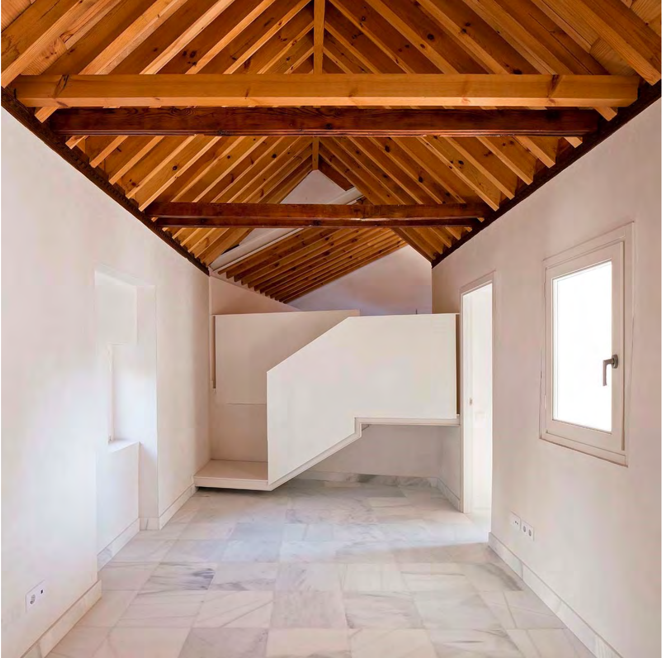
Fig. 12 – Zayas house. Interior - Source: photo of Fernando Alda
