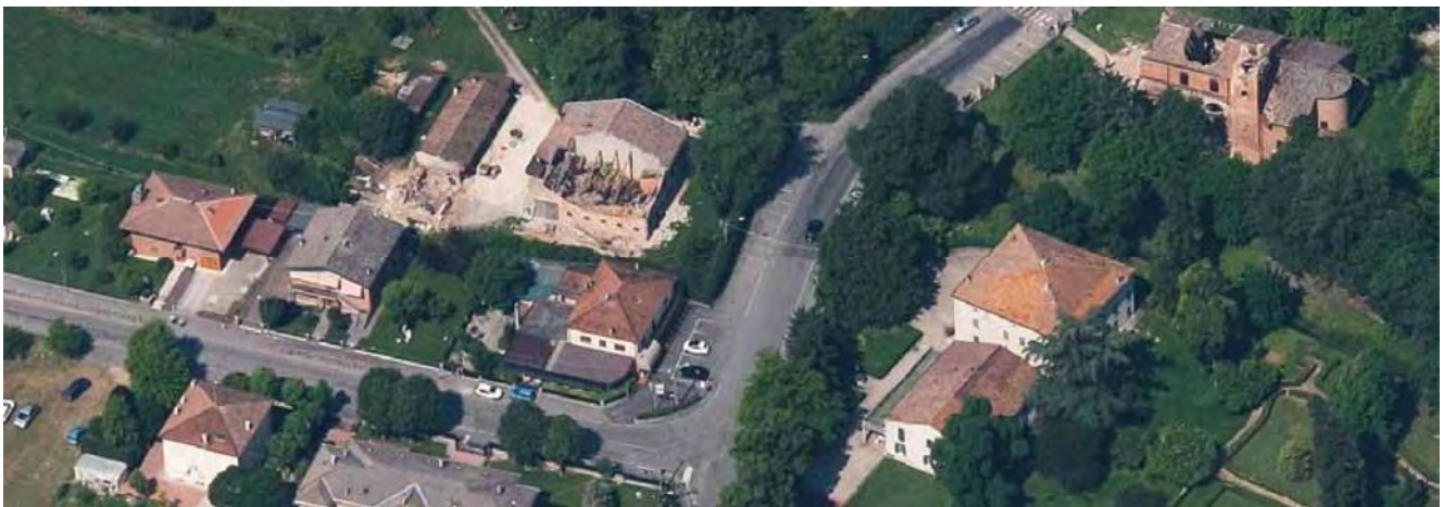
Fig. 2 – Medolla (MO), the roof, resting on long span walls, collapsed and directly contributed with its thrust to the out-of-plane overturning of the walls.
