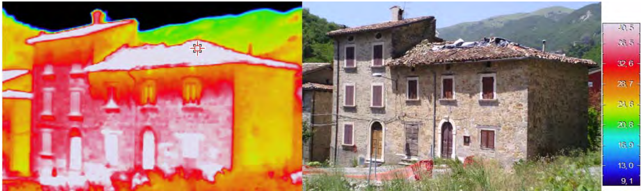
Fig. 5 – Example of thermographic tests on heterogeneous masonry (Trisungo)
