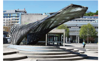
Fig. 15/ BUGA Fibre Pavilion , 2019, M. Fornes & THE VERY MANY. Fonte: Wikimedia Commons. Autore: Joachim Köhler.
