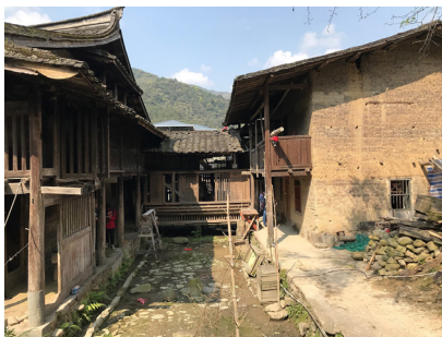
Fig. 4. View of the internal service courtyard, in which the systems of crossings, distribution by galleries and water collection are evident (photo by M. Calia, March 2019).
