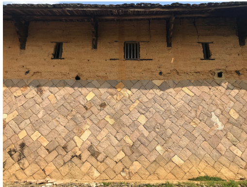
Fig. 7. Detail of a portion of the large fortified wall made of stone and rammed earth (photo by M. Calia, March 2019).
