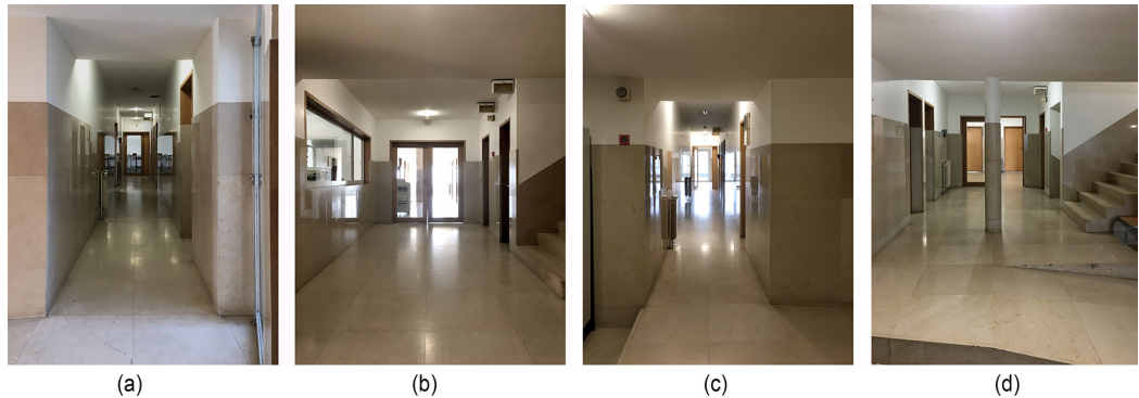
Fig. 10. The different entrances of the towers on the corridor at level 0 (photo by A. Castro).
