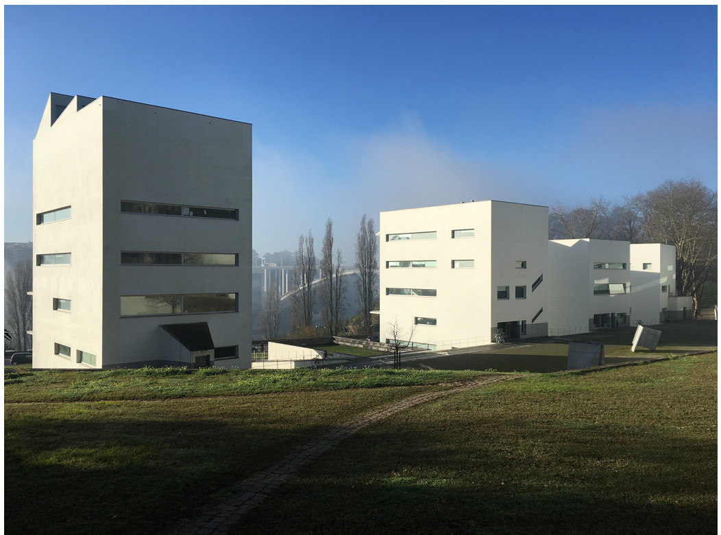
Fig. 9. View of the towers overlooking the access courtyard (photo by A. Castro).
