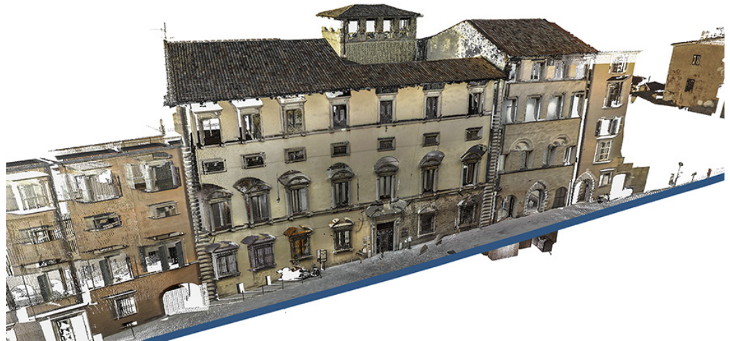
Fig. 4. Result of the integration of the pointcloud taken by laser scanning and the one of the rooftop obtained by photogrammetric drone acquisition.
