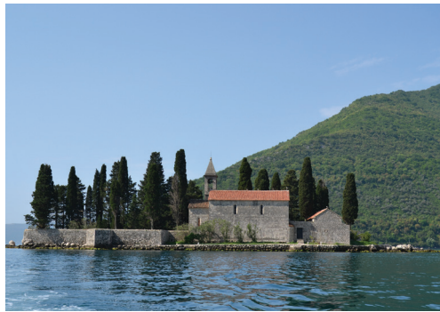
Fig. 5. The island of St. George in Croatia. Drawing of the island and general plan of the monastery (above); view from the sea (bottom).
